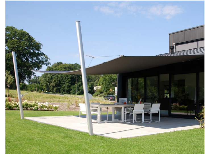
Tensile fabric canopy on ground screws.
